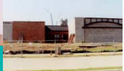
Below, Norick Art Center construction
